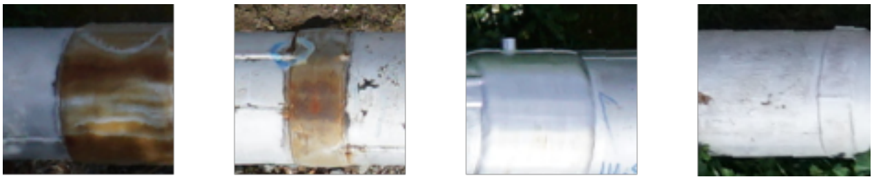
Figure III – Remediation repairs on pipes
