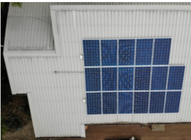
Figure 3 – Bird's eye view of a pitched roof. The area further from the camera becomes more difficult to view with an increased pitch and roof size.
